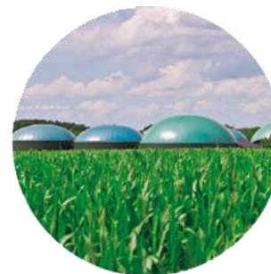
Energy from Chemical Fuels
